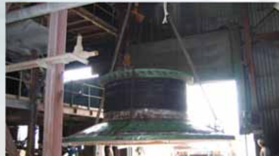
100 ton ball mill in Alaska
