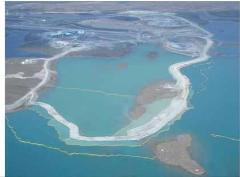
Bay Goose Dike Construction July 21 2010
