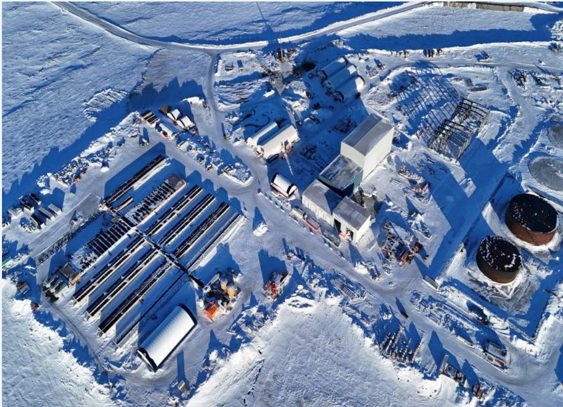
◆ Goose Project Camp Construction Area, February 2024
